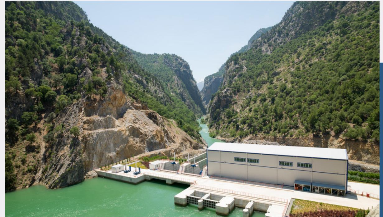
Starting operation in 2013, Kuşaklı HEPP is located in Adana, on the Seyhan River. The plant has twin Tiger turbines, each with a 10-MW capacity, and a total installed capacity of 20 MW.
