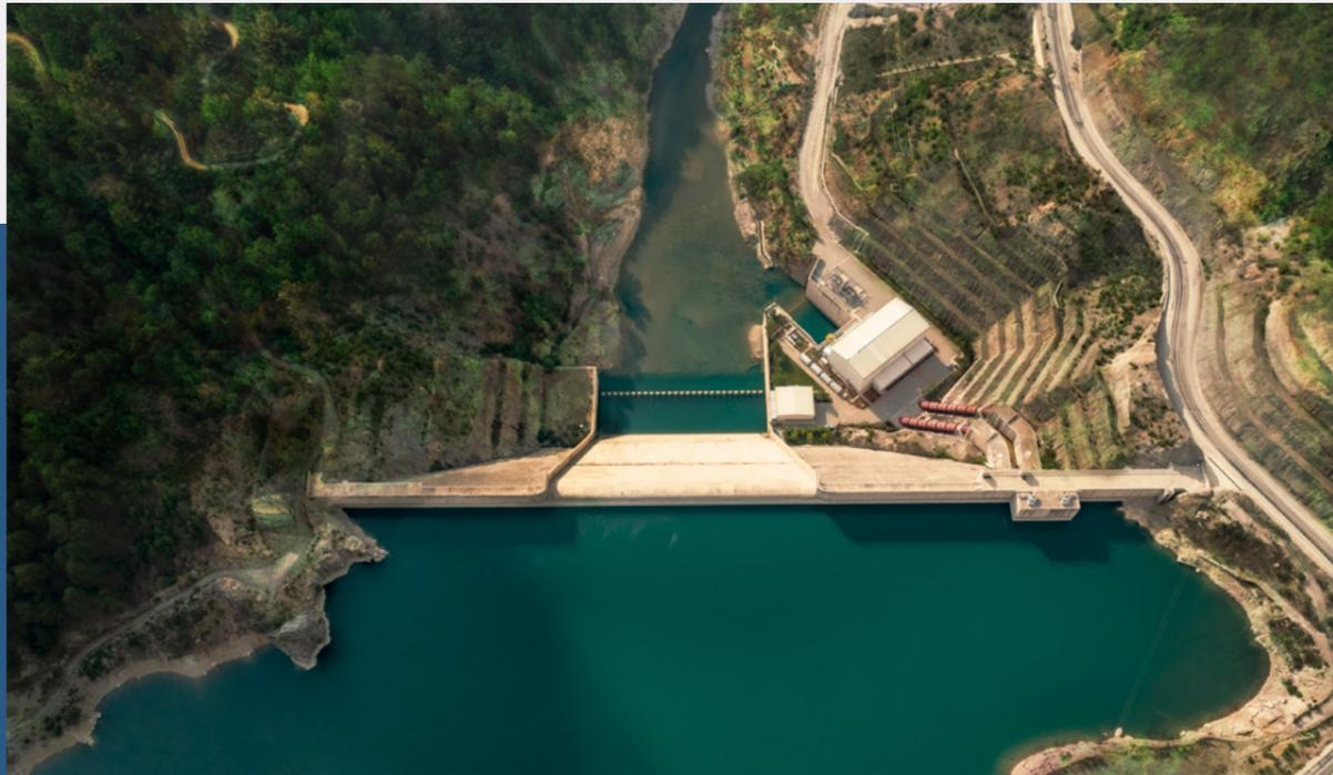
Starting operation in 2013, Köprü HEPP is located in Adana, on the Göksu Bayou of the Seyhan River. The dam has an RCC body and twin Francis turbines, each with a 78-MW capacity. Its total installed capacity is 156 MW.
