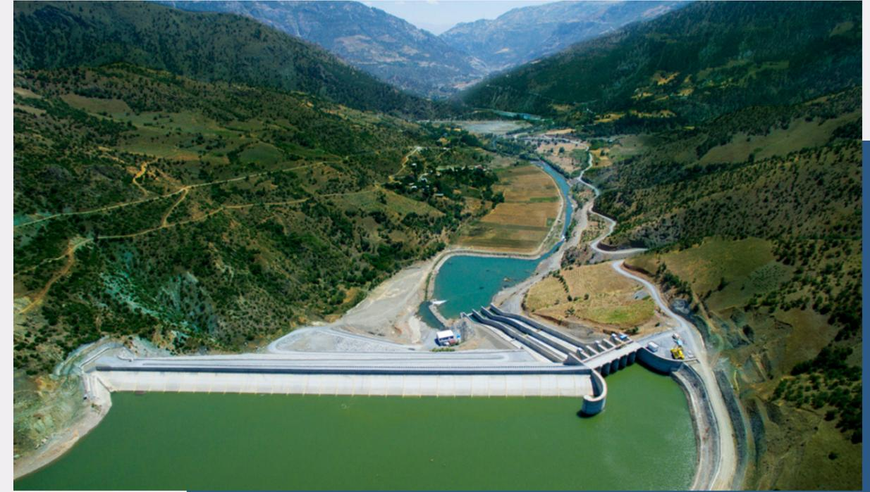
Starting operation in 2013, Sarigüzel Dam and HEPP is located in Kahramanmaraş, on the Ceyhan River. The project, which is filled with sand, gravel and rock, has a concrete-covered front and two Francis turbines, each with a 49-MW capacity.
