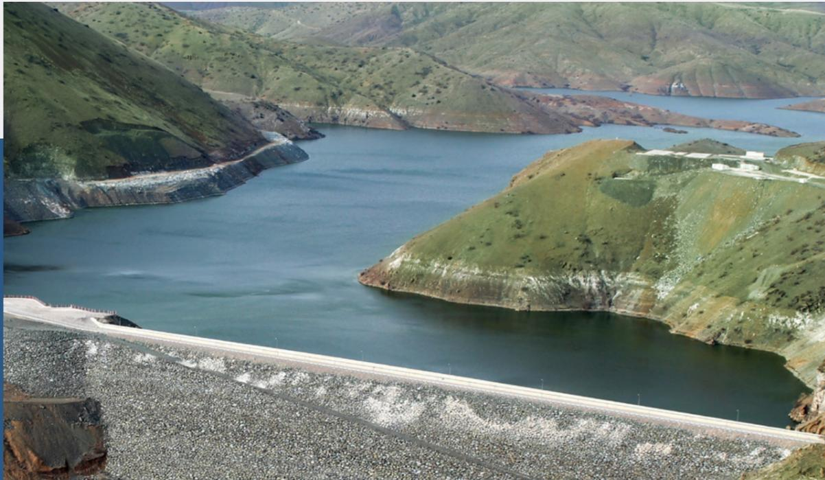
Starting operation in 2014, Kandil Dam and HEPP is located in Kahramanmaraş, in the Ceyhan Basin. The project, which includes a rock fill dam with a concrete-covered front, has a total installed capacity of 208 MW. Its two Francis turbines have a 102-MW capacity and its single environmental turbine has a 4-MW capacity.
