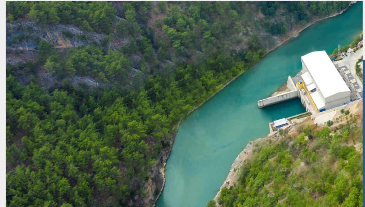
Starting operation in 2014, Kavşak Bendi HEPP is located in Adana, on the Seyhan River. The rock fill plant with a concrete-covered front has the highest installed capacity on the Seyhan River. It has three Francis turbines with a 62-MW capacity and a single environmental turbine with a 5.4-MW capacity.
