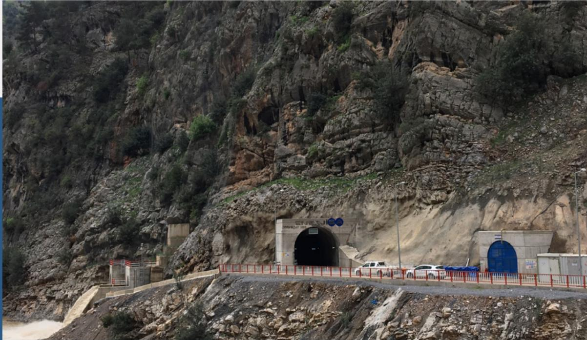
Starting operation in 2017, Doğançay HEPP is located in the Seyhan Basin, Adana, on the Doğançay Creek. This plant, which has a capacity of 62 MW, is built using a tunnel boring machine (TBM) instead of traditional methods. All of the plant's units are subterranean, except for the regulator area.
