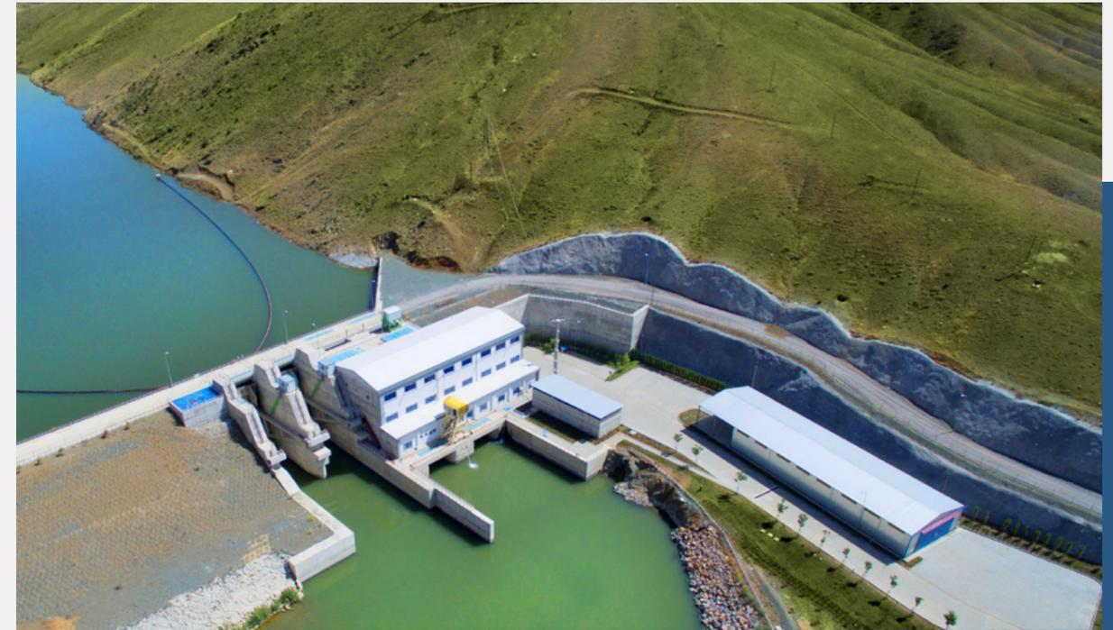
Starting operation in 2013, Dağdelen Regulator and HEPP is in Kahramanmaraş, in the Ceyhan River Basin. The plant has two tiger turbines, each with a 4-MW capacity.
