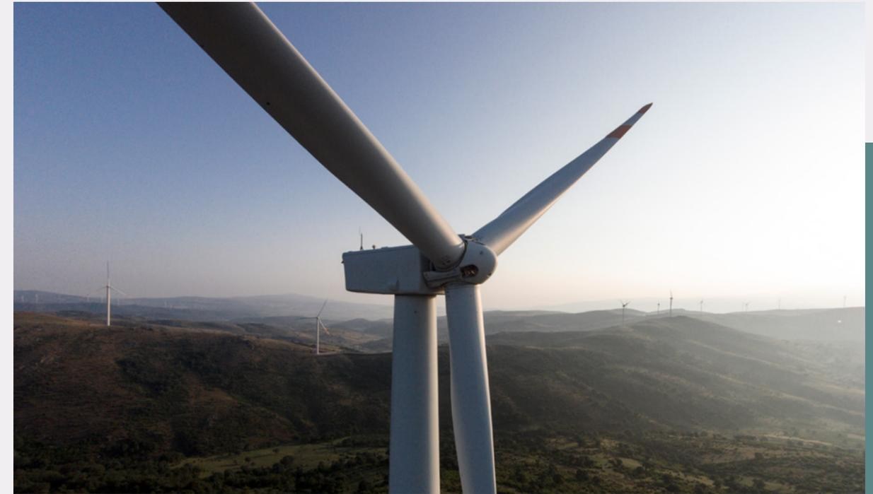
Starting operation in 2013, Balıkesir WPP is located in Balıkesir and has a capacity of 143 MW with 52 turbines. The plant is connected to the TEİAŞ' Poyraz and Balıkesir 154-kV switch. The project was awarded the "Carbon Gold Certificate" by The Gold Standard Foundation.
