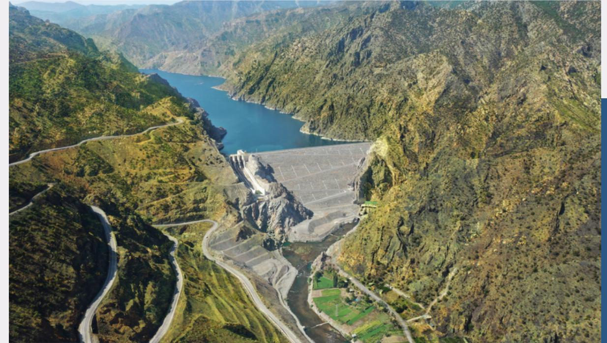
Starting operation in the second quarter of 2014, Arkun HEPP is located on the Çoruh River on the provincial border of Erzurum-Artvin. The plant's total installed capacity is 245 MW with three main turbines with a 78-MW capacity and two environmental flow plants with a 5.4-MW capacity.
